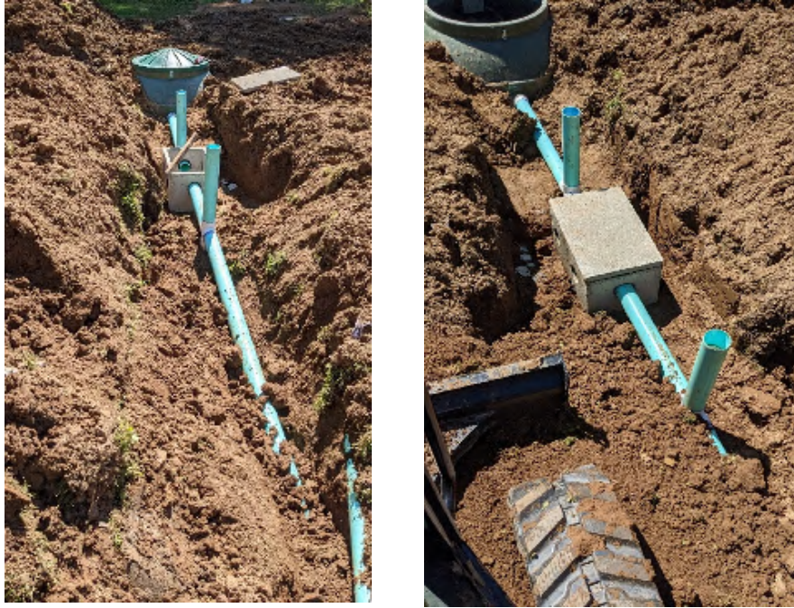
Figure 1. Examples of completed septic replacement.
